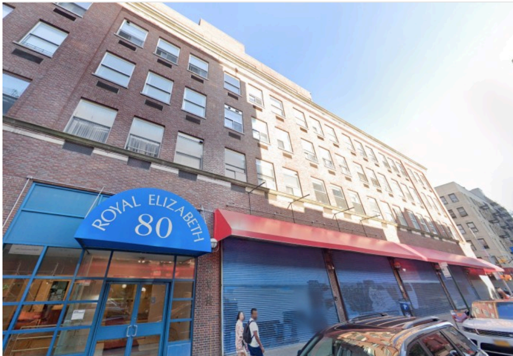
80 Elizabeth Street (Credit - Google)
